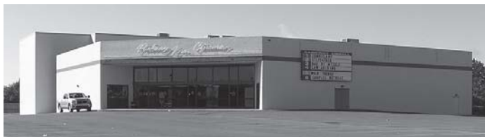
PARKWAY – Exterior of the Parkway in Natchitoches, LA. Refurbishment of the lobby, common areas and two of the original auditoriums will be completed by May 1st.
